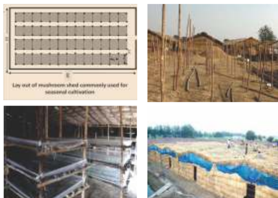
Fig.43: Lay out and different steps in the construction of hut
