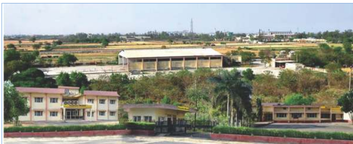
Fig. 21: Aerial view of HAIC Agro Research and Development Centre, Murthal
