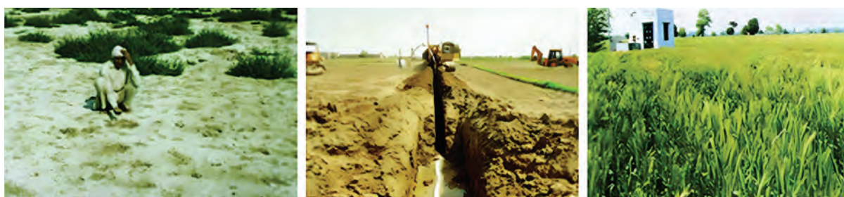
Fig. 1.5 Highly saline soil (left), mechanized laying of subsurface drainage (middle) and bumper crop of wheat in the reclaimed land
